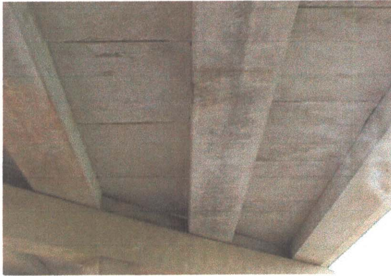
BOTTOM OF DECK
