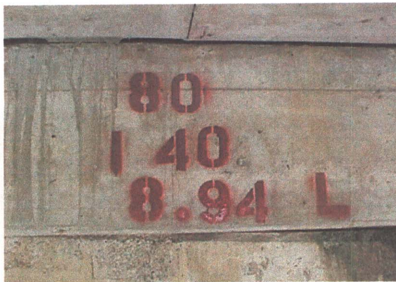
BRIDGE NO. AT ABUTMENT # 1
