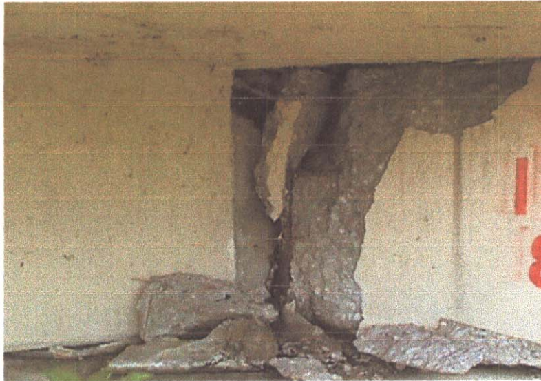
BREAKOUT W/EXP. REBAR L.S. ABUT-1
