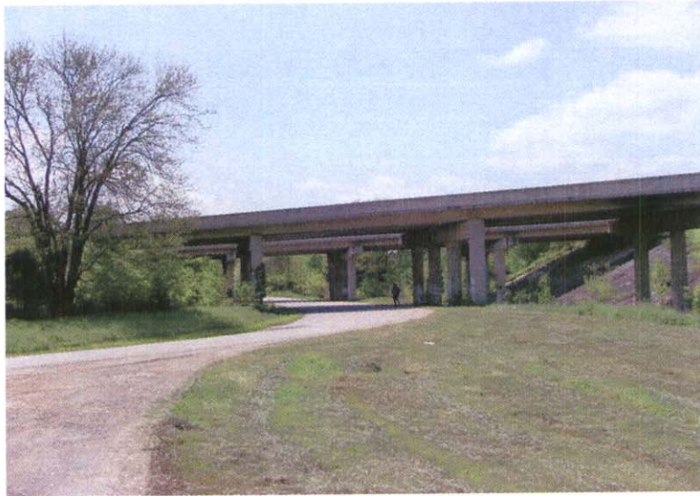
LEFT SIDE VIEW @ UNDERPASS
